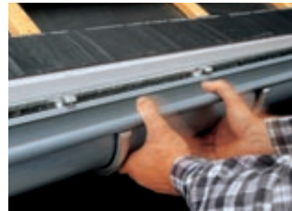
Step 3: The RHEINZINK® gutter is snapped into place securely and permanently.
