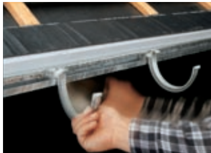
Step 2: Gutter brackets are locked into place with a simple twist.
