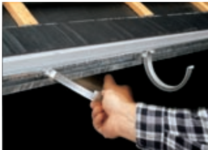
Step 1: Snap-lock gutter brackets are inserted into the mounting rails in the rafter area.
